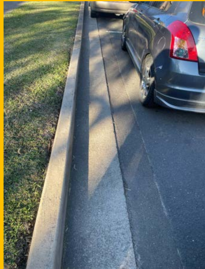
No. 016: 75m. Repairs to road surface at kerblin
