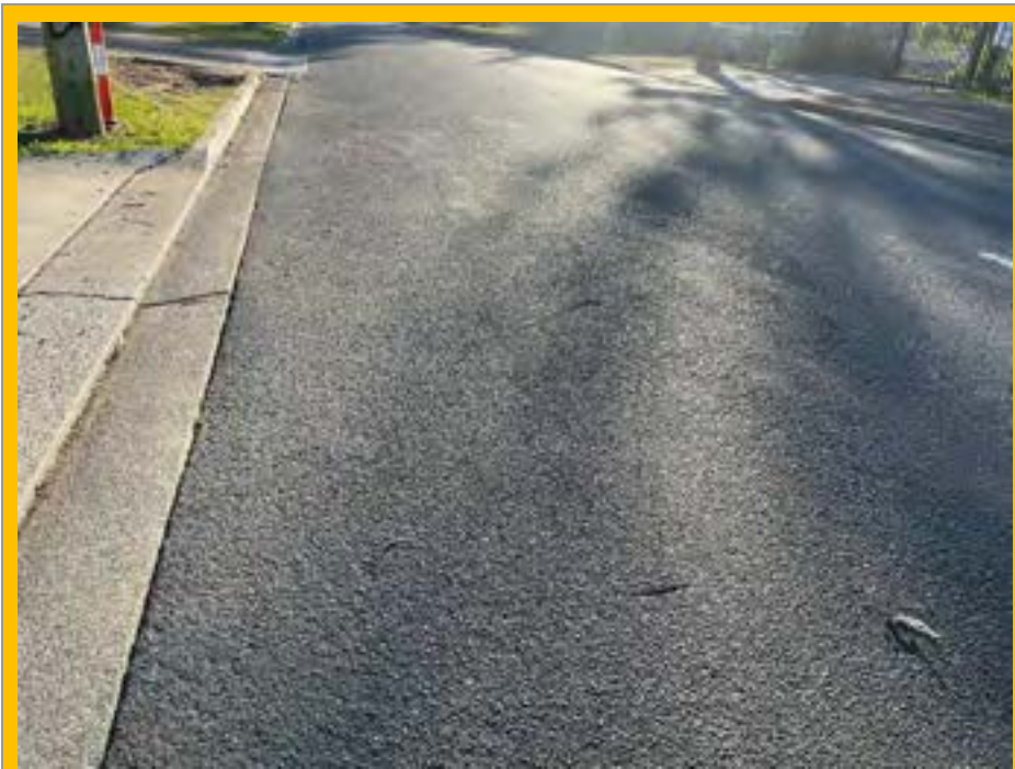
No. 017: varying gouge marks from 85-90m
