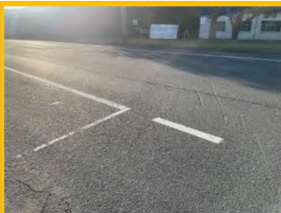
No. 065: gouging toward road centreline at eastern layback to 24 Harris St (approx. 274m)
