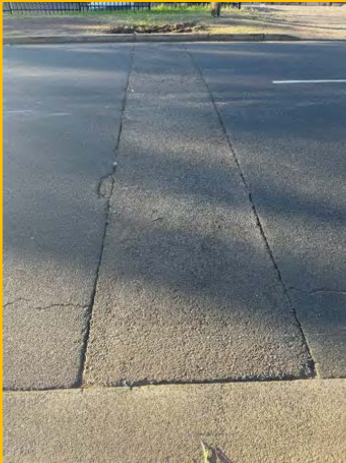
No. 015: repairs to road surface across width of street at approx. 78m
