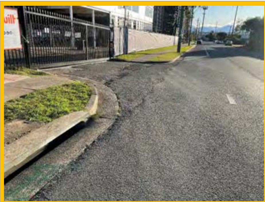
No. 092: overview of entry to the at grade station car park
