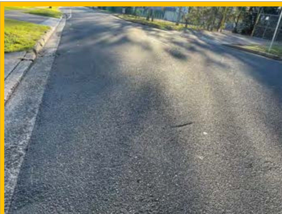
No. 038: 180m. gouge marks at layback to 12 Harris St extending to road centre
