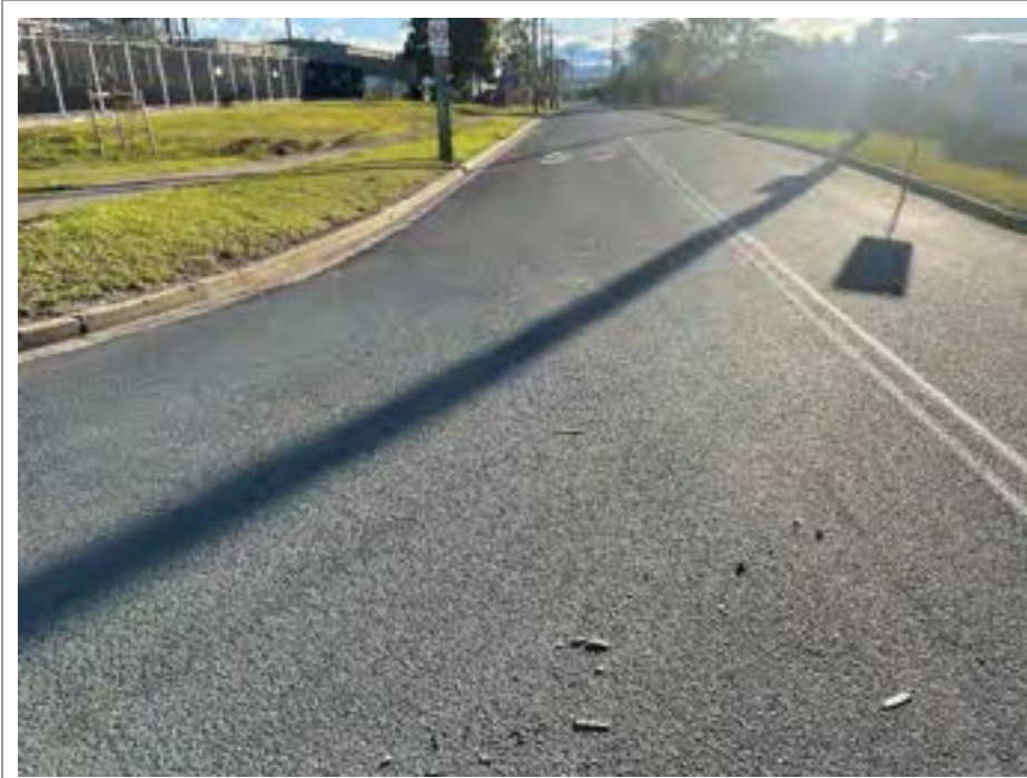
No. 001: Overview of Harris Street from the southeast corner at the intersection to Glossop Street. Survey began from this corner at 10m intervals which are marked for distance reference.
