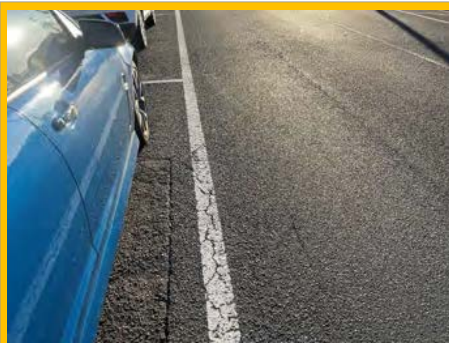
No. 125: 520m. repairs to road surface in parking bay
