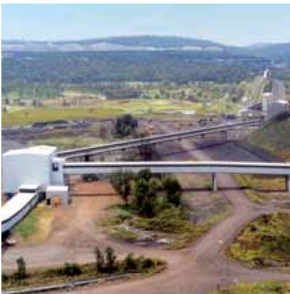
Callide 'C' Coal Handling Plant
