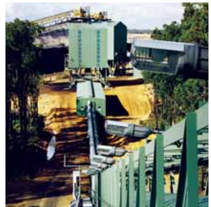
Premier Mine to Collie Overland Conveyor
