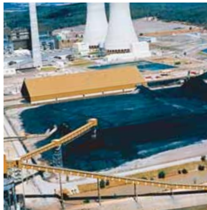
Mt Piper Coal Handling Plant
