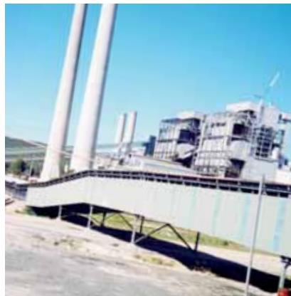
Wallerawang Coal Handling Facilities
